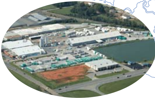
★ PipeLife Plant Siloam Springs, Arkansas
