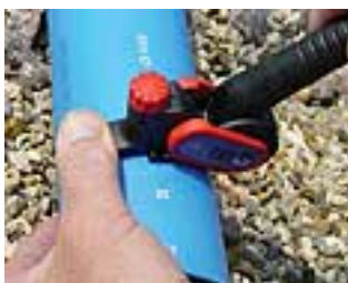
Rotate the peeling tool keeping a firm grip with the thumb, and peel around the pipe.
