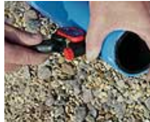
Using small pumping movements bring the peeling tool down to the mark.
