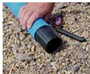
Exposed internal layer ready for scraping and welding.
