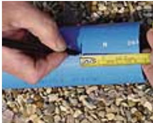
Measure and mark the pipe.
