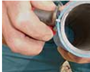
Insert the blade between the outside and internal layer.
